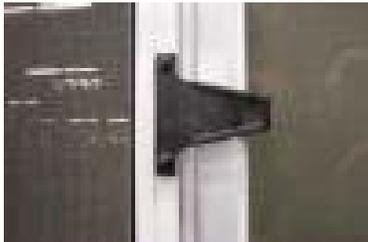
The latch is attached to the screen mullion with two rivets. Carefully center punch the rivet heads. Using a suitable power drill bit, drill off the rivet heads. Carefully remove the rivet shaft with a nail or drift punch.
