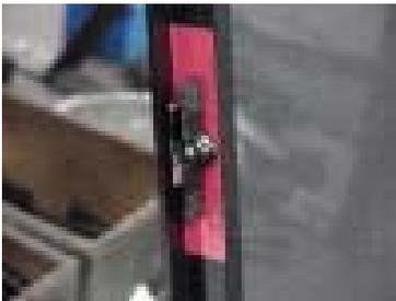
Each latch is attached to the vent frame with a screw through a nylon sleeve in the center. The sleeve keeps the screw from backing out as the latch is opened and closed. Remove the screw with a suitable Phillips
