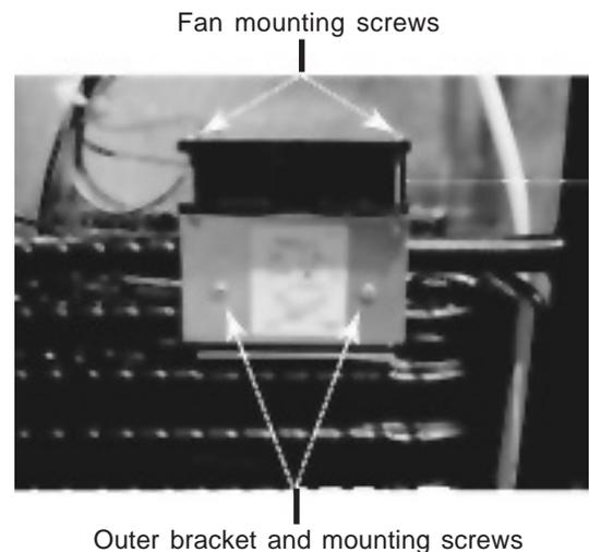
Figure 24. Fan Mounted on Top of Absorber Coil.
