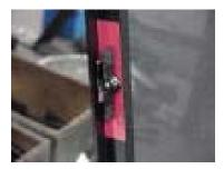
Each latch is attached to the vent frame with a screw through a nylon sleeve in the center. The sleeve keeps the screw from backing out as the latch is opened and closed. Remove the screw with a suitable Phillips
