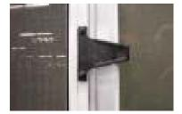
The latch is attached to the screen mullion with two rivets. Carefully center punch the rivet heads. Using a suitable power drill bit, drill off the rivet heads. Carefully remove the rivet shaft with a nail or drift punch. Discard the damaged latch. Place the new latch and align the holes.
