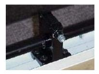
Crank the window open to give yourself working room. Remove the crank screw and crank. Remove the screen. Remove the four screws holding the operator. Lift up the operator. This will take the tension off the torque tubes, which can then be taken out of the operator.
